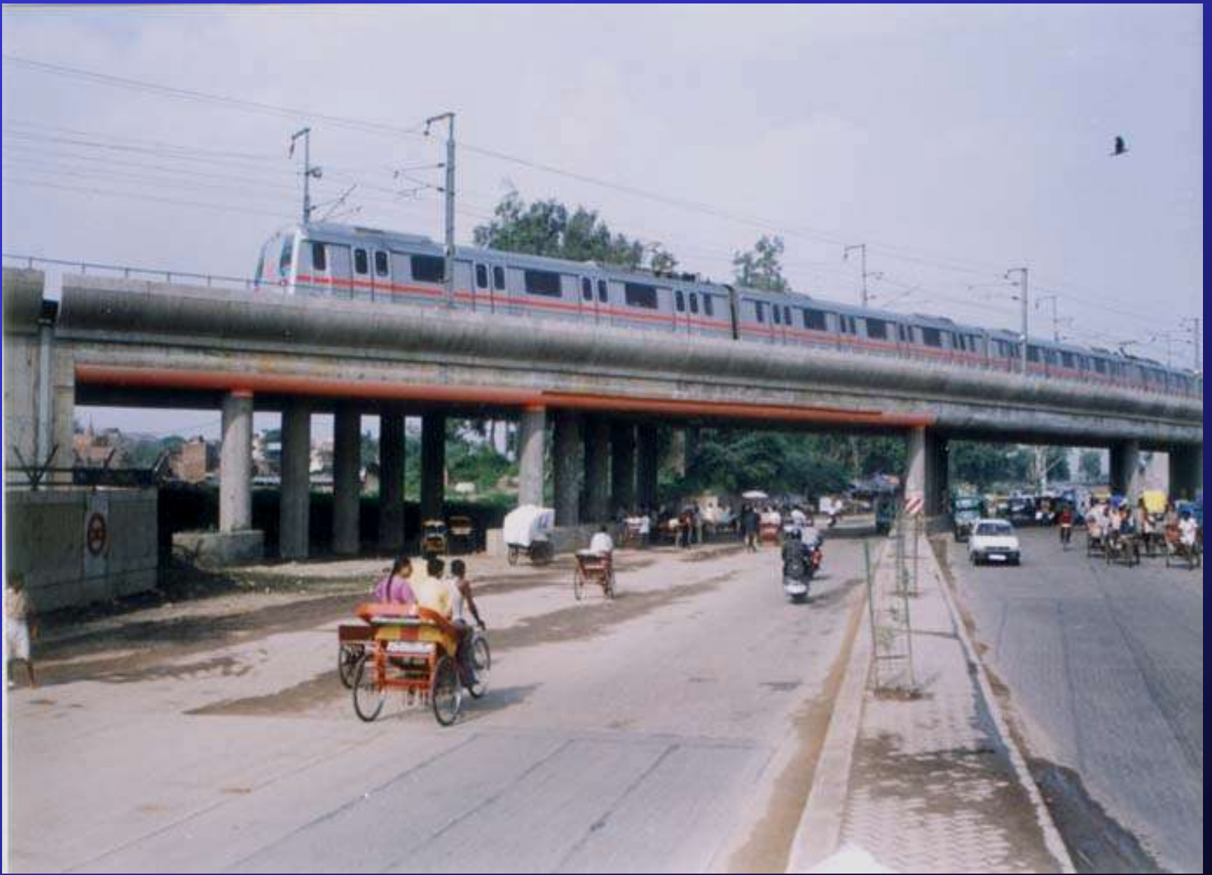
G. T. Road Fly over - Integral Bridge
